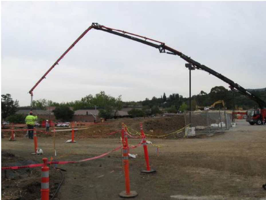
Figure 4. Cement truck pouring cement with a hydraulic arm (photograph by Peter Y. Chou).
