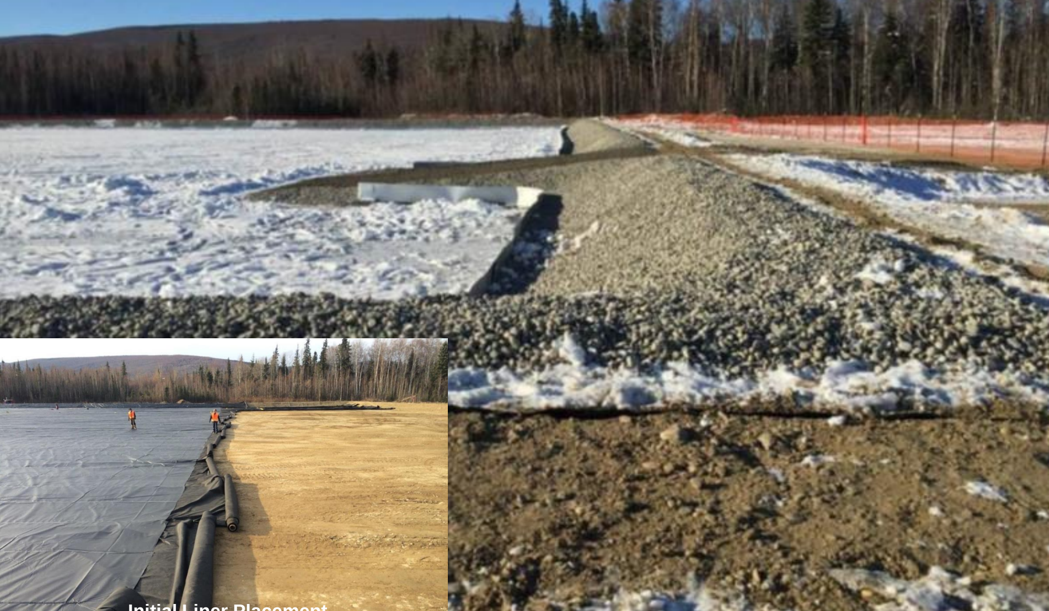
Initial Liner Placement
