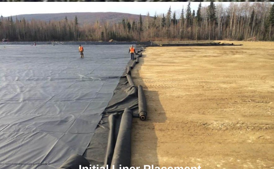
Initial Liner Placement
