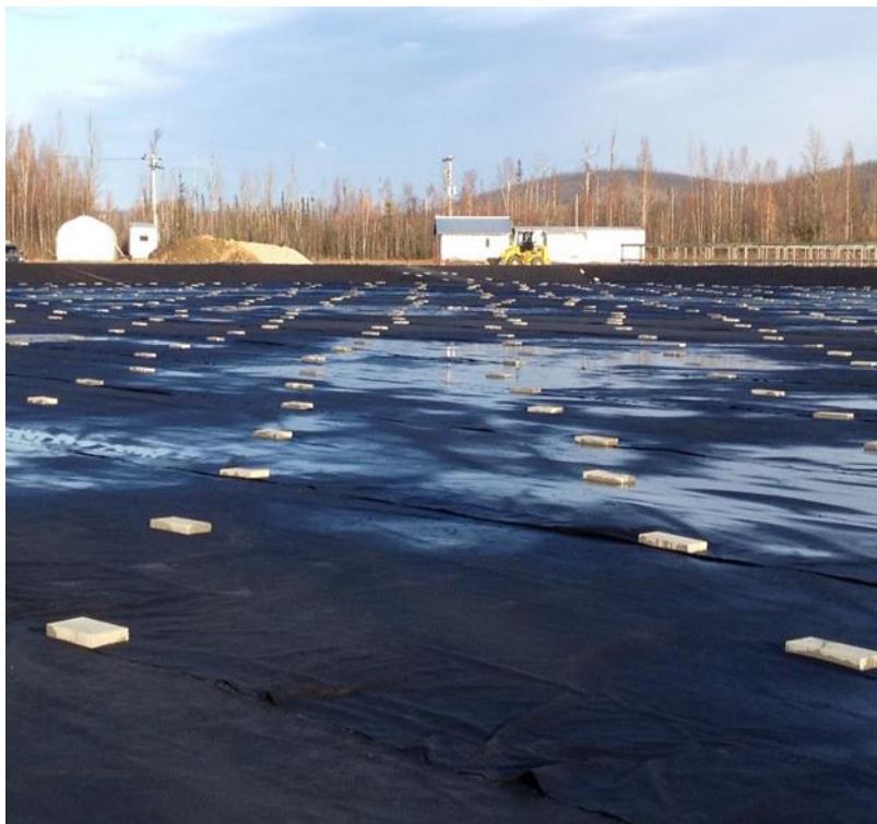
Figure B-6: Concrete Paver placement over Liner/Geofabric
