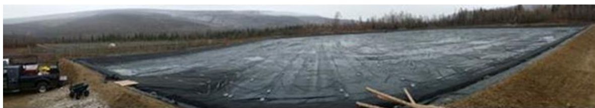
Figure E-4: Panoramic View of Finished Herder Test Basin with Liners and Geotextile Installed
