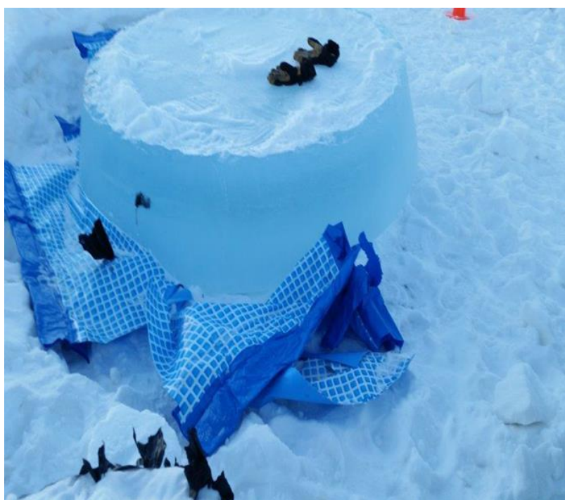
Figure B-11: 8 Foot diameter 'iceberg' post form removal
