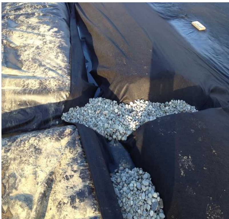
Figure B-5: Keyway with Liner and Geofabric and Rock Armor to Stabilize prior to backfill
