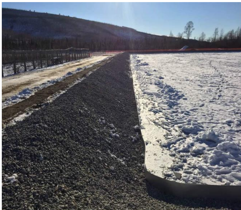
Figure B-8: Rock Armor and Flashing installation along southern side of Test Basin
