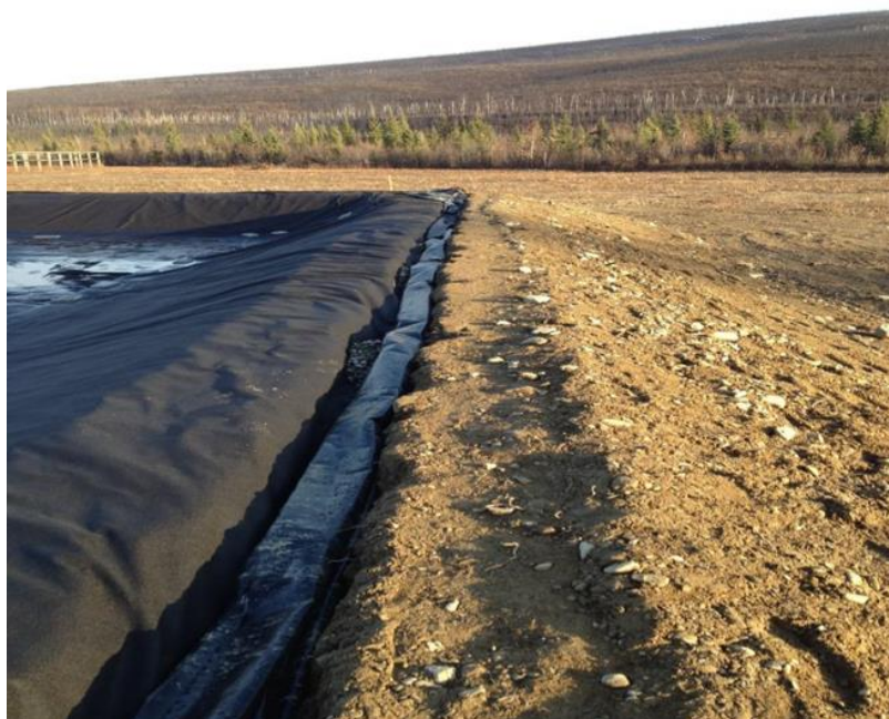
Figure B-4: Keyway Liner and Geofabric Installation
